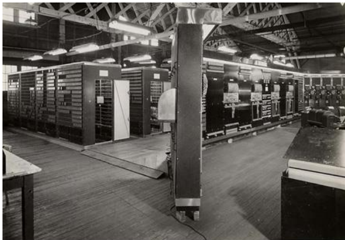
Mark II, general view of calculator frontpiece, 1948.
